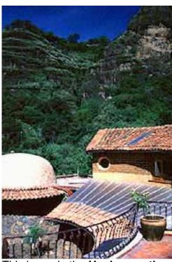
This home in the **Huehuecoytl eco village** (Eco village house) is made largely from natural materials, much of them from on-site. Harvested Rainwater supplies a cistern, which supplies super-efficient fixtures with water pre-heated by the sun, which drain through a greywater system, which waters fruit trees that shade the house in summer, reflect sun onto the house in winter, block cold wind, and supply fruit.
